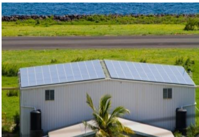
Figure 17: PV Panels for SWRO System
