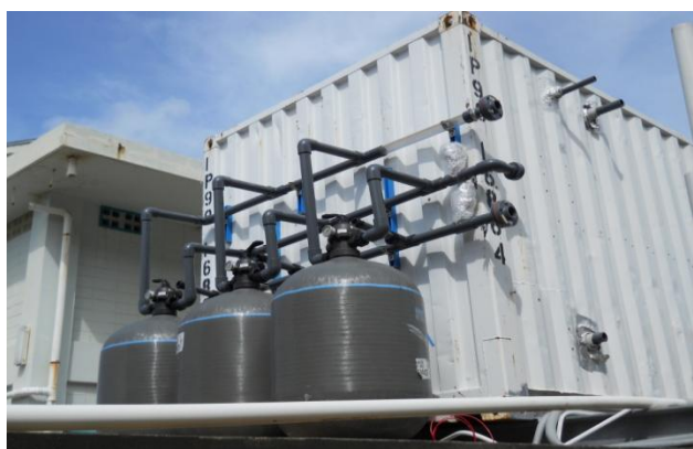
Figure 13: Reservoir Tanks
