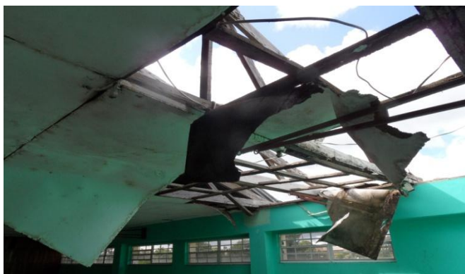
Figure 31: Marchand Community Centre Dilapidated Roof
