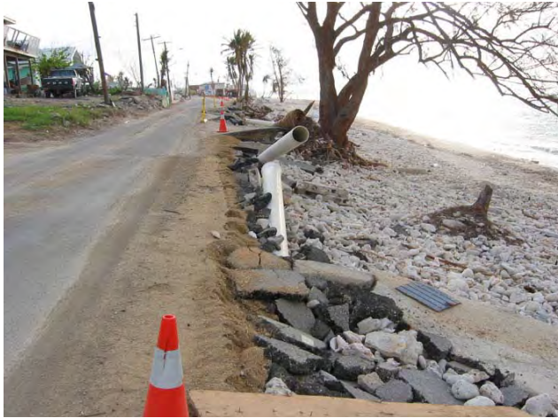
Photo 10. Water lines along coastal road exposed and damaged by hurricane Ivan. Credit: ECLAC 2005
