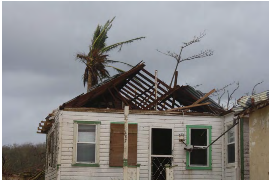
Photo 1 Roof damaged Caymanian-style home from Hurricane Paloma, Cayman Brac, November 2008. Credit: Unknown
