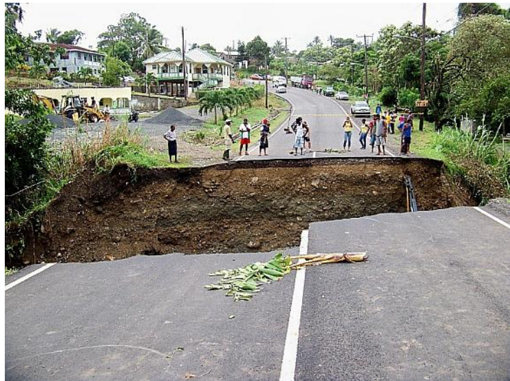
Figure 8: A collapsed road from Hurricane Tomas' torrential rains Source: http://www.djmrp.com/slu-crisis/slu-crisis-hurricane-tomas.htm
