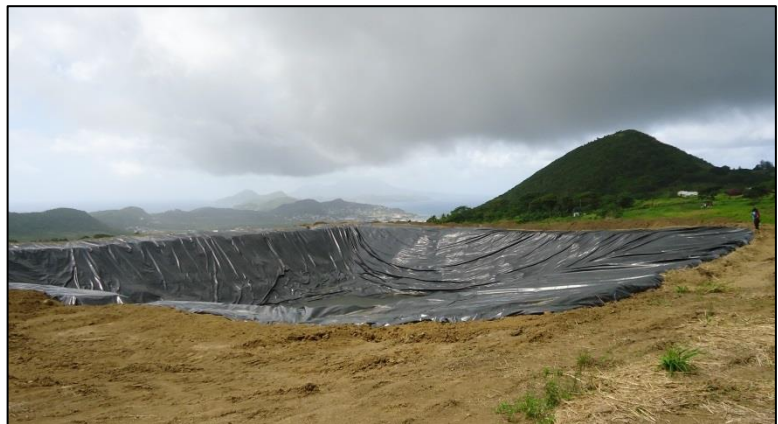
Figure 5.2: Water Catchment Dam being constructed to supply small farmers on Stapleton Estate, St. Peters
