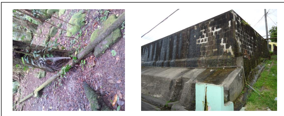
Figure 4.4: Leakage in Distribution Network and in Existing Storage within Reservoirs
